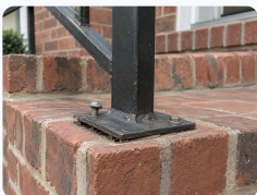
Building B stair, second landing Sep 29, 1:47 PM UTC
